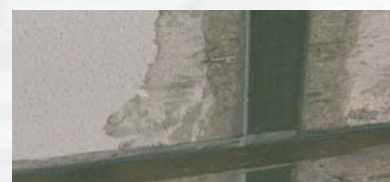
Detail CFK-Lamelle
