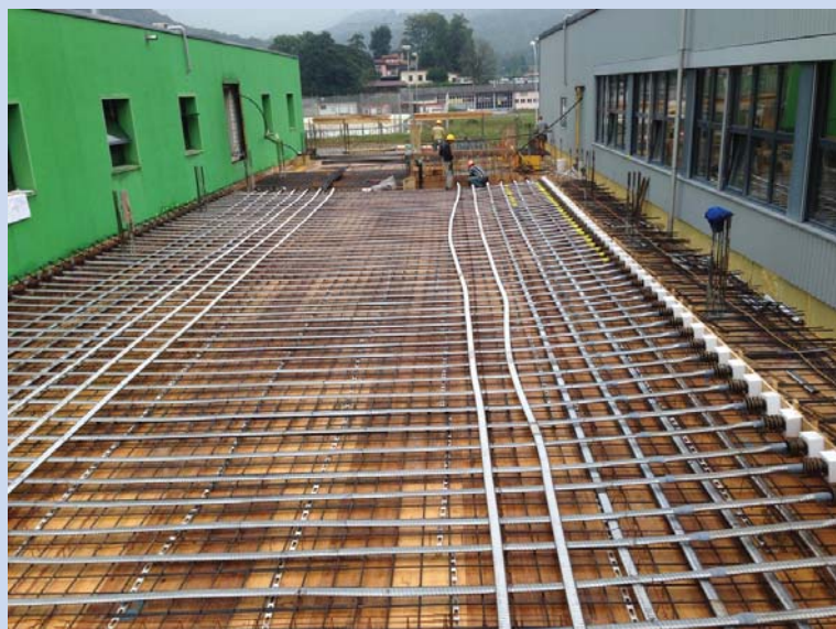
Cavi posati, teste mobile in sagex
