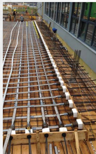
Cavi posati, teste mobile in sagex
